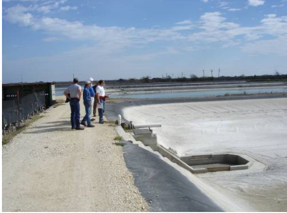
Figure B10a: Reclamation and FWS staff inspecting lined rearing pond at Uvalde NFH.
